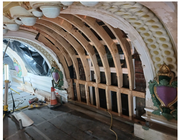
Reconstruction of the Lancashire Panel
