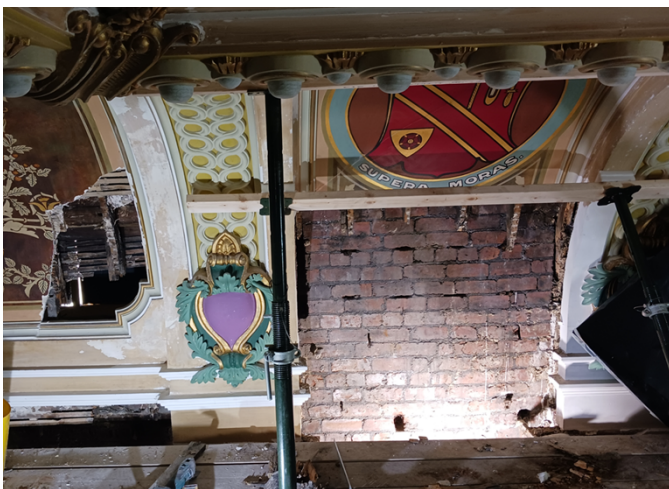
Partial Removal of Panels 1 and 2
